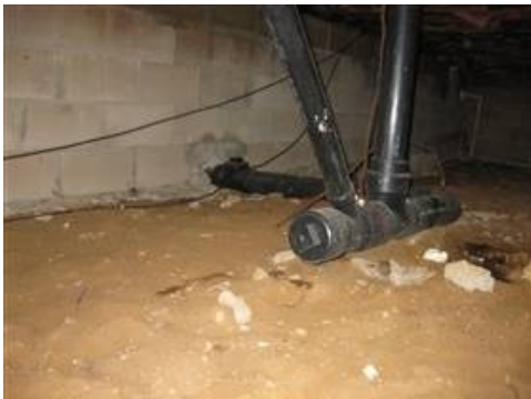
Photo X-5 Sewer cleanouts in crawl space
