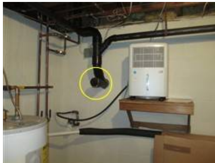
Photo X-8 Main sewer cleanout
