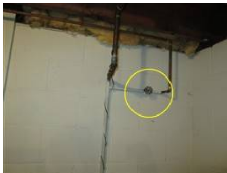
Photo X-6 shutoff for front hose bib
