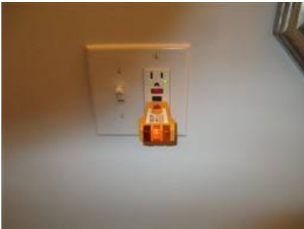
Photo 23-1 Basement powder room
