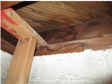
Photo 43-1 Basement - front wall
