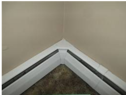
Photo 43-2 Area above front basement wall
