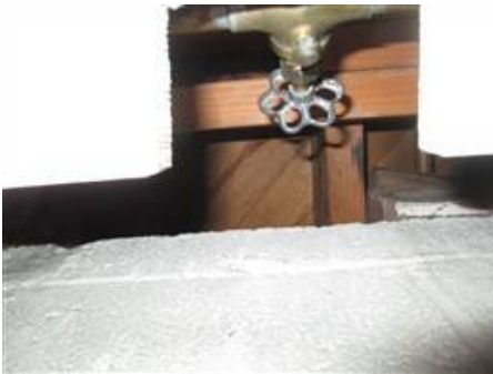
Photo X-5 Front hose bib shut-off in wall above water meter
