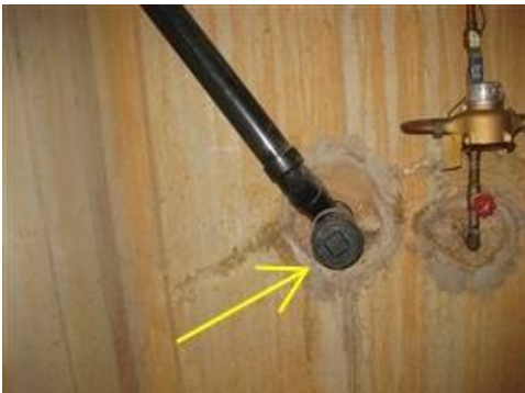
Photo X-3 Sewer cleanout
